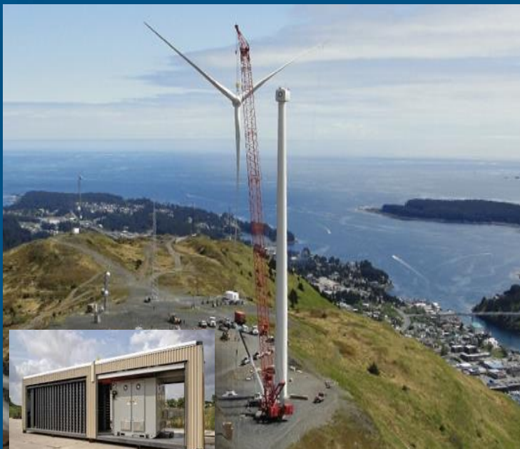
Kodiak has achieved 97% renewable penetration with hydro-wind-battery-flywheel system (above)
