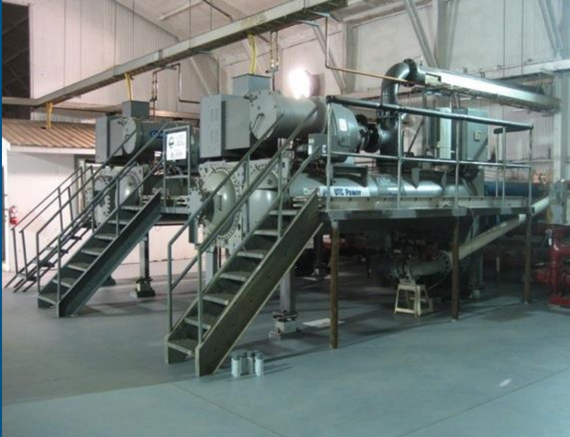
400 kW Power Generation from ORC with 72 C
