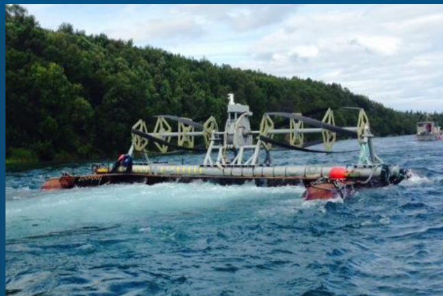
Hydrokinetic turbine installed the community of Igiugig (above)
