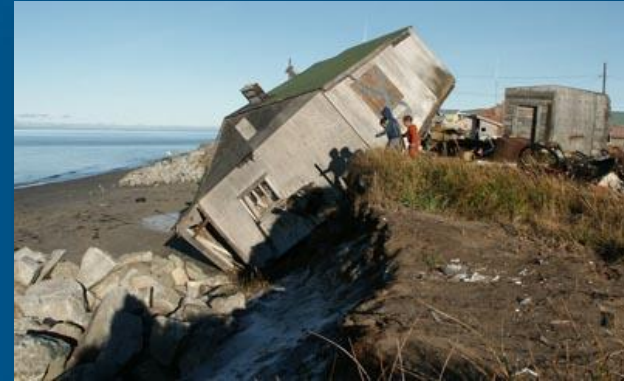
Erosion from fall storms - Shishmaref
